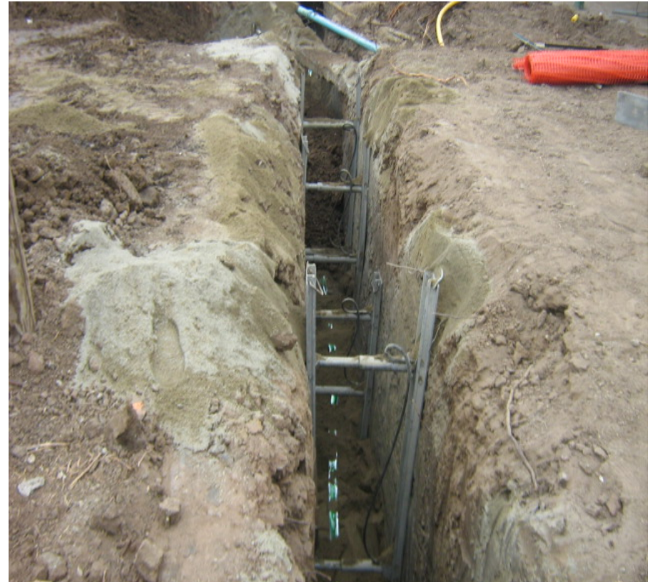
New Utilities Trenching (Shoring per OSHA)
