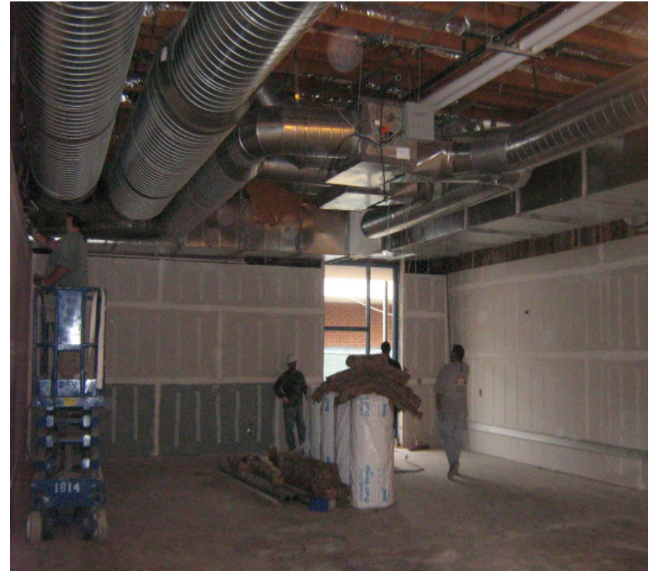
New Classroom HVAC Duct Work & Drywall
