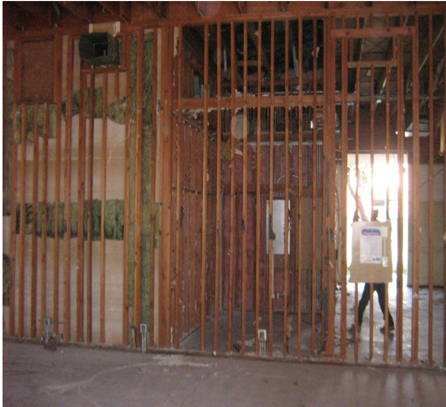
Classroom Building Demo
